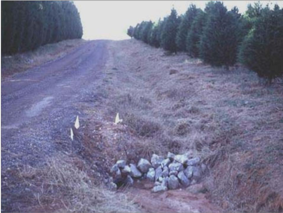
Rip rap will slow water down and cause swirling in front of the rock which may help settle soil or it may cause a wash in front of the rip rap depending upon the velocity of the stream. Therefore several rows of rip rap would be required on steep slopes.
