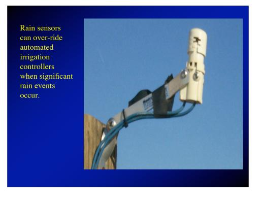
Rain sensors on automated landscape irrigation systems are mandatory in some communities. Likewise, rain over ride sensors should be installed on automated nursery irrigation systems. The notches at the top of the sensor can be set to over ride irrigation system after  $\frac{1}{2}$  inch or 1 inch of rain fall.
