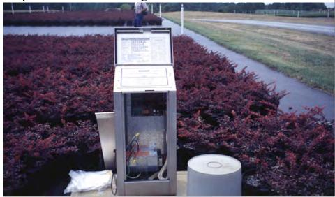
Cycled irrigation is the use of multiple irrigation cycles of irrigation compared to one long irrigation cycle. Automated controllers and electric solenoids are required for cycled irrigation, since turning manually operated valves multiple times over many irrigation zones in a nursery is impractical. Cycled irrigation requires uniform irrigation distribution. Consequences of poor irrigation distribution are magnified when cycled irrigation is used.
