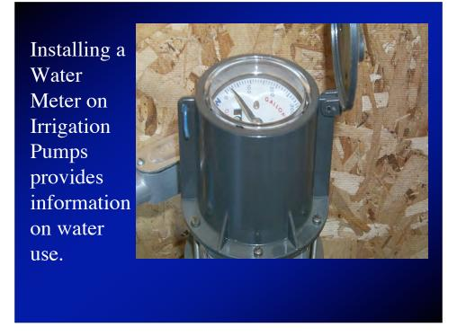
Water meters are not standard equipment on most nursery irrigation systems due to cost. However, water meters are an excellent investment because they provide information on daily water use. Data recorded from water meters can be used to determine water applied for calculation of interception efficiency in container beds.
