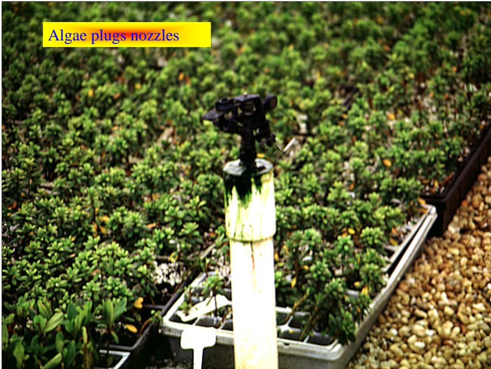
Burying or painting light exposed pvc distribution lines may be required if nutrients are contained in the irrigation water. Otherwise irrigation system filtration and disinfection practices may be required to control algae.
