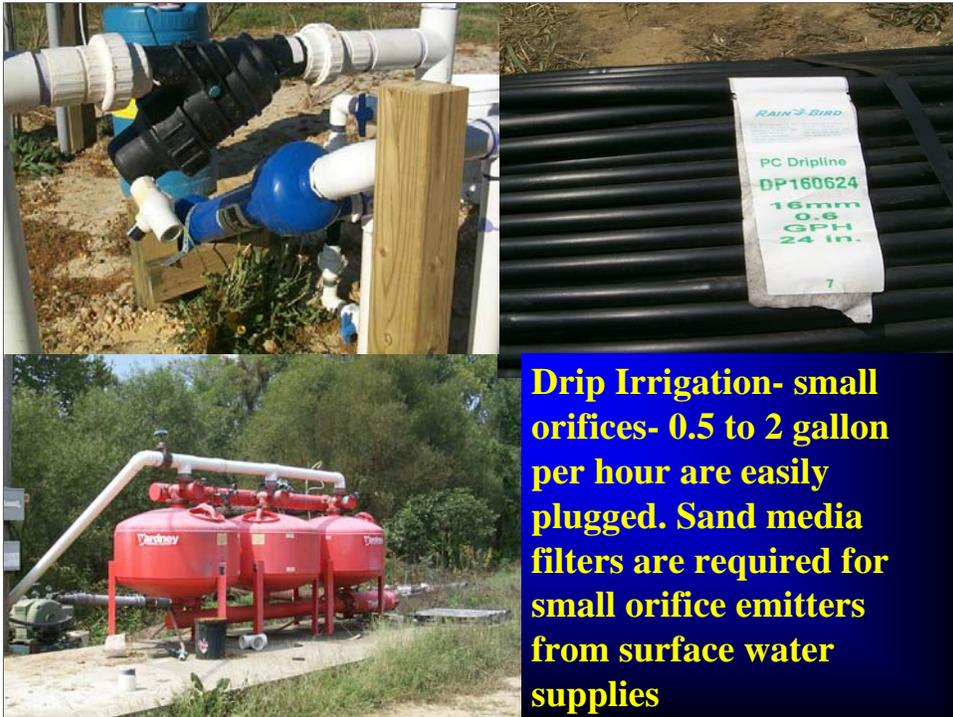
Drip irrigation nozzles have very small orifices and apply water in ranges from  $\frac{1}{2}$  gallon per hour to 2 gallons per hour (upto 5 g[h]). A sand separator and disk filter (upper left picture) may provide adequate filtration for well irrigation supplies but sand media filters (lower left) are required for irrigation from surface water supplies.
