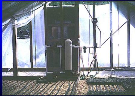
Bromine is considered to be a better algaecide than chlorine and is therefore preferred by some nurseries for propagation greenhouses. The lower picture shows a bromine injector in a greenhouse. This particular injector used bromine tablets which may no longer be available.
