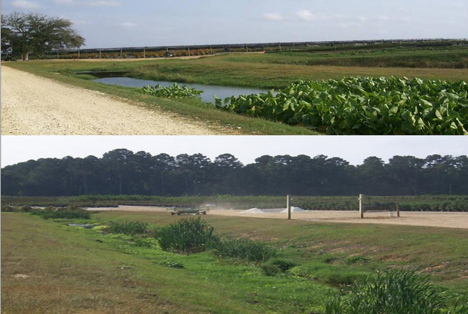
Directing runoff water through standing surface water followed by movement through aquatic plant filters removes nutrients, sediment and reduces disease organism viability.
