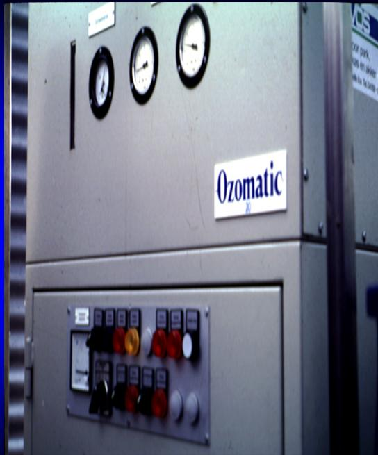
Ozone injection is also an infrequent technology used for treatment of nursery irrigation water supplies. The unit pictured above was seen in a very advanced greenhouse facility in the Netherlands. Ozone was also being used at a nursery visited in Oregon for disinfection of irrigation water used for propagation greenhouses. An Ozone test kit, much like a test kit used for testing chlorine in swimming pool water is used to determine appropriate concentrations.
