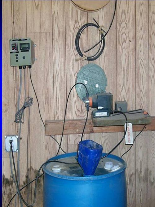
Products such as DiSolv (designed for low volume systems) or AquaSolv designed for overhead irrigation systems can be injected into water supplies as an alternative to chlorine or bromine injection. A small injection pump is used to inject low rates of these products into the irrigation system.
