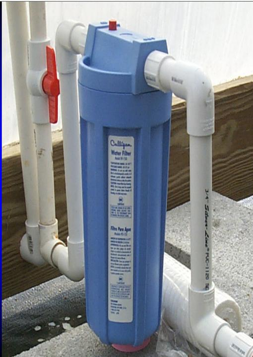
Since propagation greenhouses use relatively low volumes of water, cartridge filters with various types of cartridges may provide adequate filtration, particularly if water is pre-filtered before being pumped to propagation facilities.
