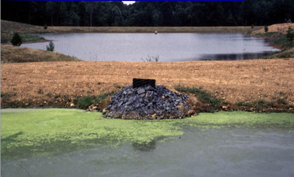
Detention structures used as a primary stage for containment of recycled irrigation supplies are very effective in intercepting nutrients, sediments and exposing disease organisms to conditions that de-activate infectious stages of the diseases.
