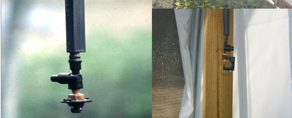
Since clog nozzles can have drastic effects on propagation facilities, adequate filtration is recommended based upon likely impurities that might cause clogging of nozzles.
