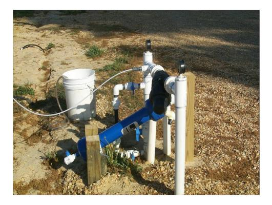
A sand separator and a screen filter are required for removing sediment from this well water supply before the water can be used in a drip irrigation system.
