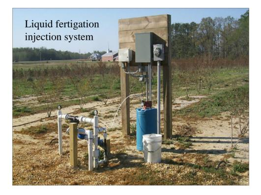
Components for irrigation of field grown nursery stock may include a well, a backflow preventer, an irrigation controller, a sand separator filter and inline screen filter, pressure gauges in front and behind filters, a fertilizer stock tank, a fertilizer injector, main lines, and distribution lines with in line emitters for application of water and fertilizers at the root zone of plants in each row.
