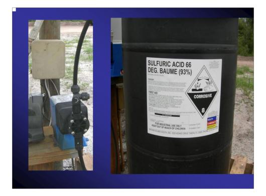
Water treatment may be required for irrigation sources that have high bicarbonates or other mineral impurities. Sulfuric acid requires injection pumps specifically designed for injection of acids. A water analysis is required to determine the amount of sulfuric acid required to neutralize the bicarbonate levels to prevent plugging of drip emitter orifices.
