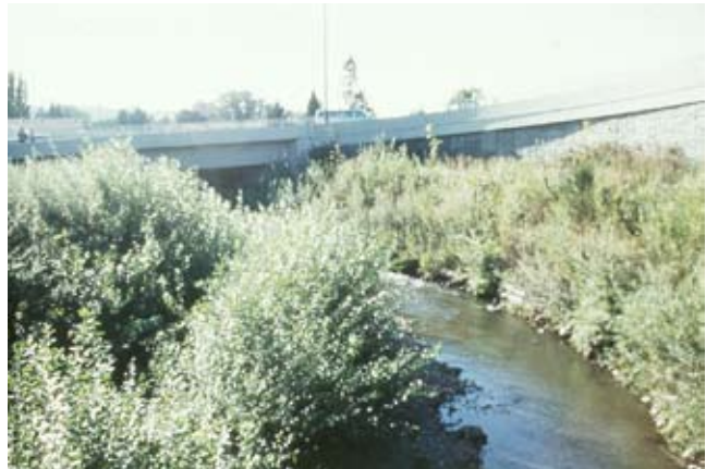
Figure TS14I-33 VRSS development after 4 years ( Photo courtesy of Robbin B. Sotir & Associates, Inc. )
