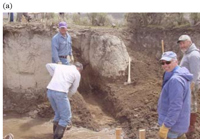
Figure TS14I-13 Brush spur being installed
