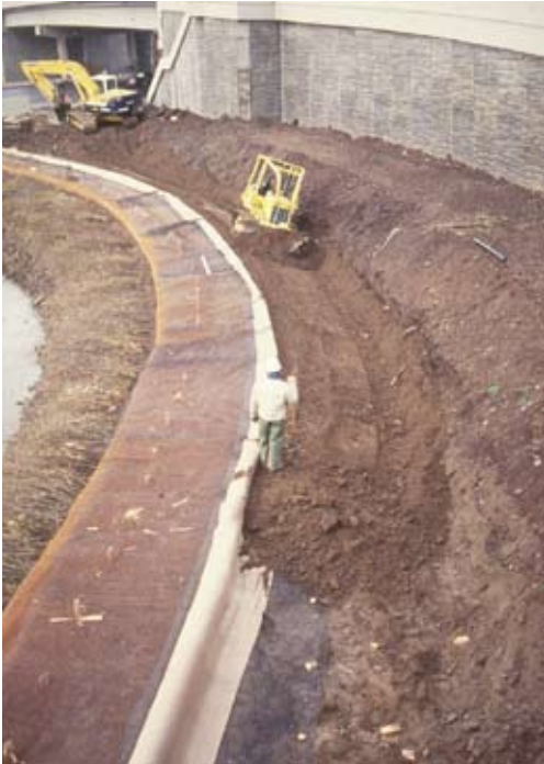
Figure TS14I-30 Fill placement within VRSS ( Photo courtesy of Robbin B. Sotir & Associates, Inc. )
