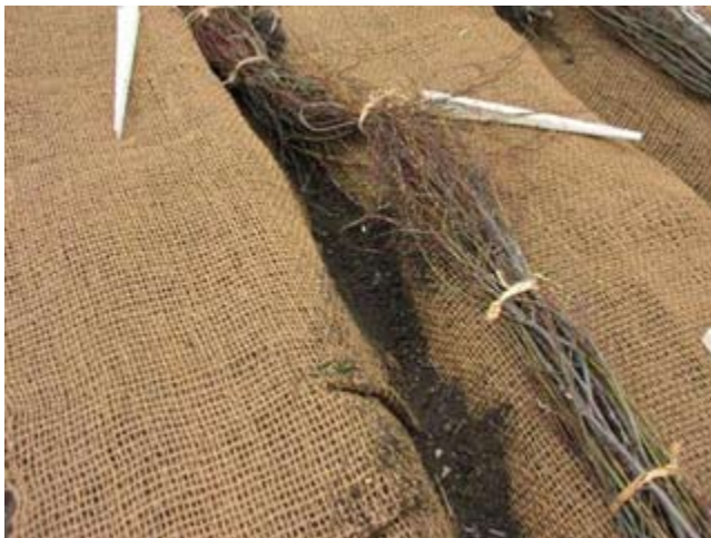
Figure TS14I-40 Combining fascines and fabric
