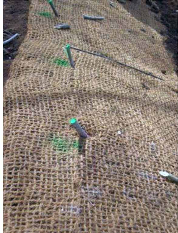
Figure TS14I-39 Live cuttings installed in fabric
