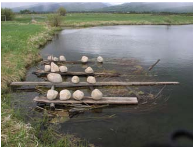
Figure TS14I-46 Soaking willow cuttings at Fox Creek, Driggs, ID
