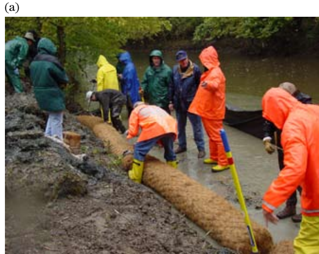
Figure TS14I-8 Installation of coir fascines: (a) Anchoring; (b) Tying of the coir fascines together ( Photos courtesy of Robin B. Sotir & Associates, Inc. )
