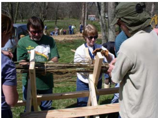
Figure TS14I-18 Assembling fascines
