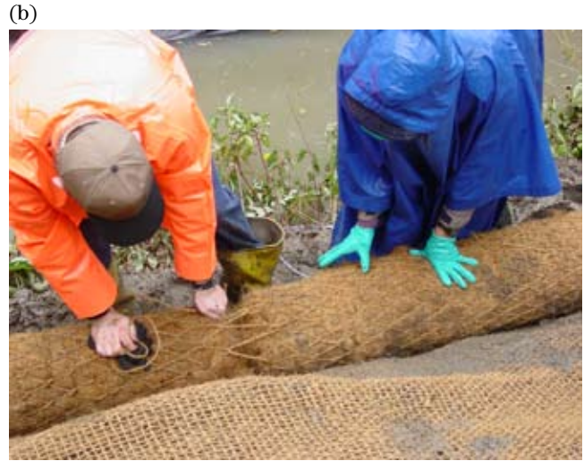
Figure TS14I-8 Installation of coir fascines: (a) Anchoring; (b) Tying of the coir fascines together ( Photos courtesy of Robin B. Sotir & Associates, Inc. )
